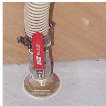
Thru-hull fitting open
